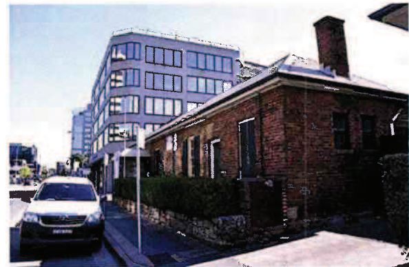
9. Introduced windows to east wall.
