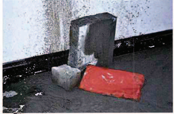
3. Removed section of concrete slab and Fortecon.
