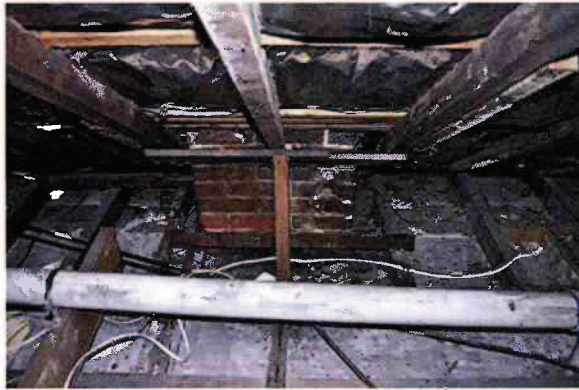
4. East chimney suspended on steel angle.
