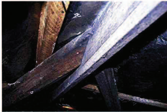
6. Rafter/ ridge board junction- drawn wire nails.
