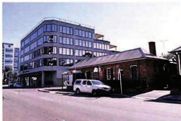
8. The subject building from the south-east.
