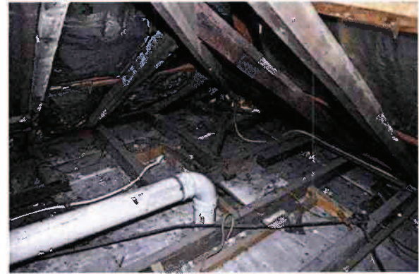
7. Eaves/ hip board framing.
